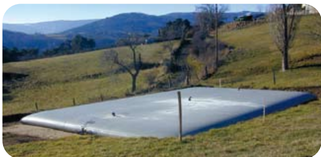
Stockage 200m3 eaux blanches
